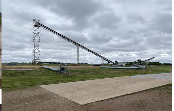
Electrical Building, (3) 100-bu pits, (2) MASABA 20,000 bph conveyor
